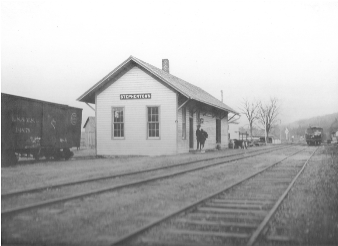
The Stephentown railroad station along the Corkscrew line of the Lebanon Springs Railroad.
